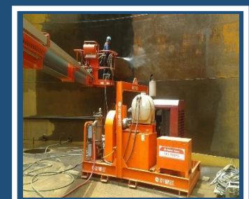
UHP Machine - Site Picture
