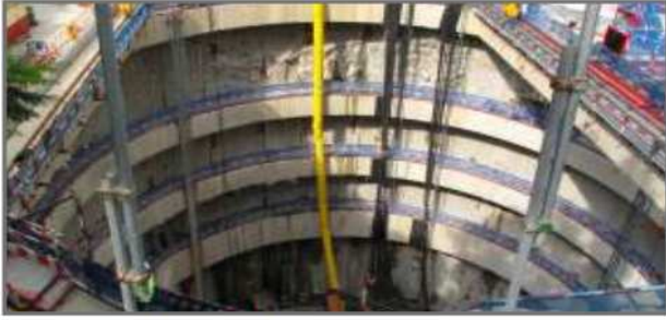
Underground construction de-watering
