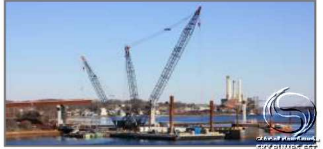
Bridge construction de-watering
