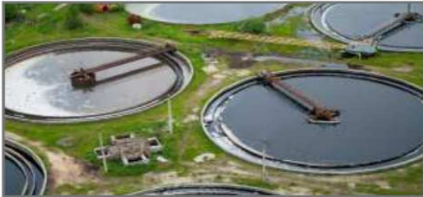
Waste water treatment plant
