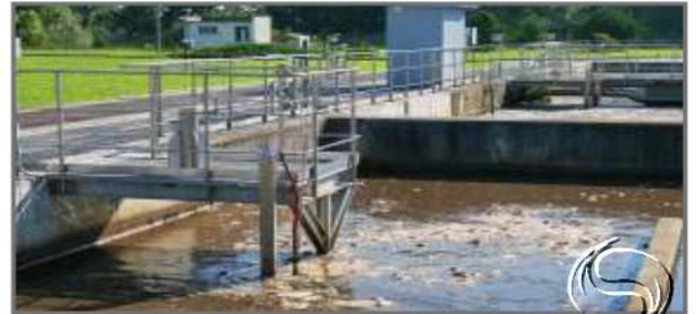
Waste water treatment plant
