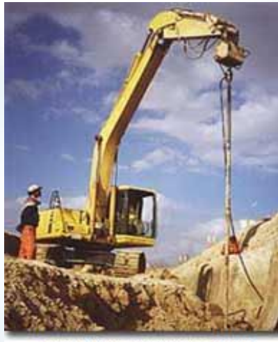
130mm Dia. x 7.5 metre Depth One Stroke. DTH Rock Drilling
