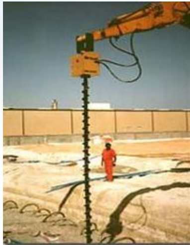
130mm Dia. x 6 metre Depth. One Stroke. Dewatering
